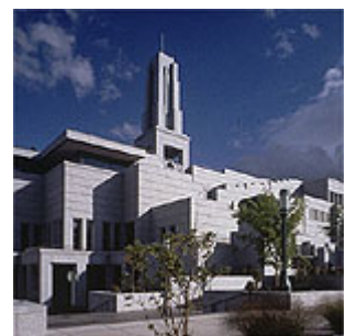
The panels of granite that cover the exterior were quarried near the source of the granite used for the Salt Lake Temple.
