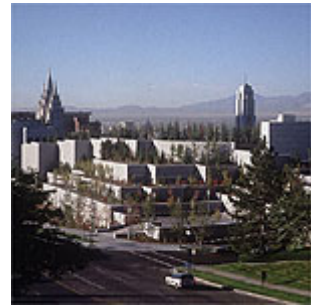
The terraced roof of the new conference center of the Church of Jesus Christ of Latter-day Saints, designed by the Zimmer Gunsul Frasca Partnership. Photo: Timothy Hursley
